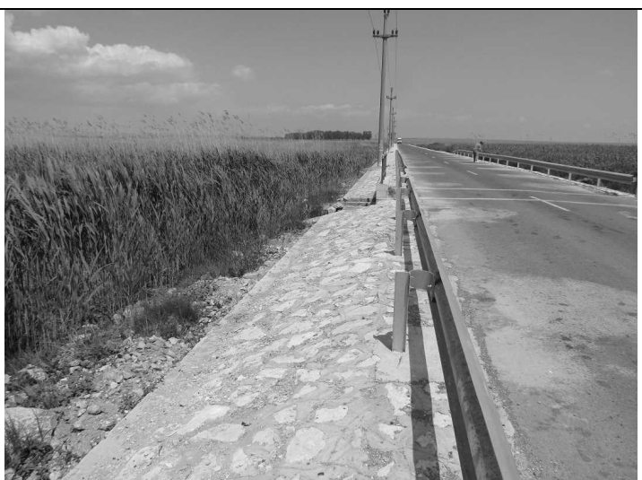
Fig. 4. Metal fence and concrete embankment along the road-sector (between Sarichioi and Enisala) with roadkillings.
